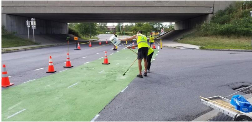
Work has begun on the first on-street, two-way *protected* bike lane in the region. Ridge Road in Lackawanna is getting a bike-friendly makeover, with the installation of a 1.4-mile protected bike lane.
